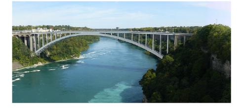
(c) A parabolic arch bridge (The parabolic arch is in compression)
